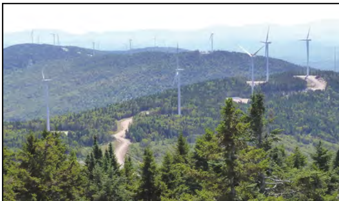
33-turbine (99 MW) Granite Reliable Power wind farm in Dixville and Millsfield, N.H.
